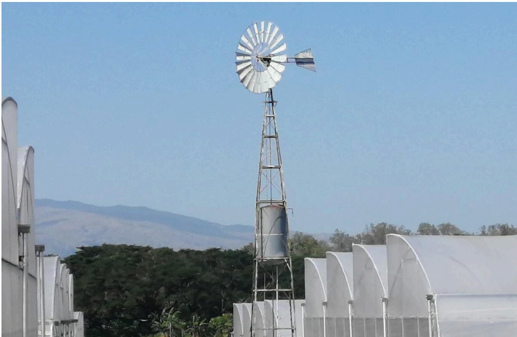
Figure 6.5.4k. Windmill driven pumps with elevated water tanks.
