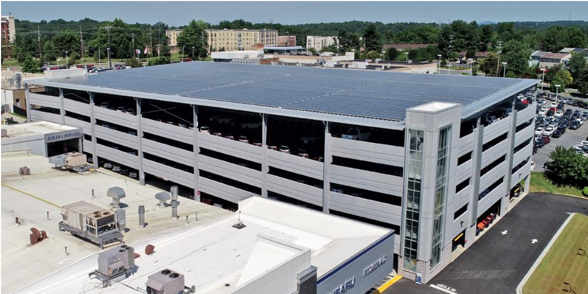
Figure 3-14: Fitzgerald Parking Garage Solar Canopy Building
