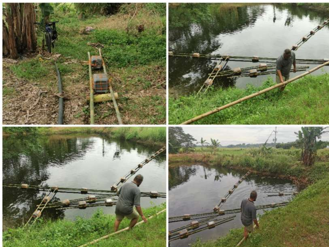
Figure 52. Construction of Bamboo Frames and Assembling the Fish Cage in the pond
