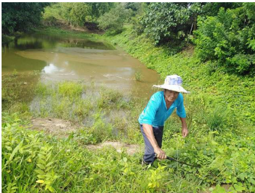
Figure 2. Removal of vegetation on SFR site at Brgy. Labney San Jose, Tarlac
