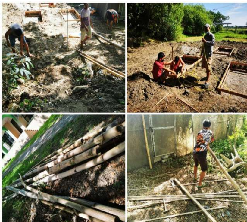
Figure. 43-46. Duckweed area selection Building and construction of duckweed artificial pond.
