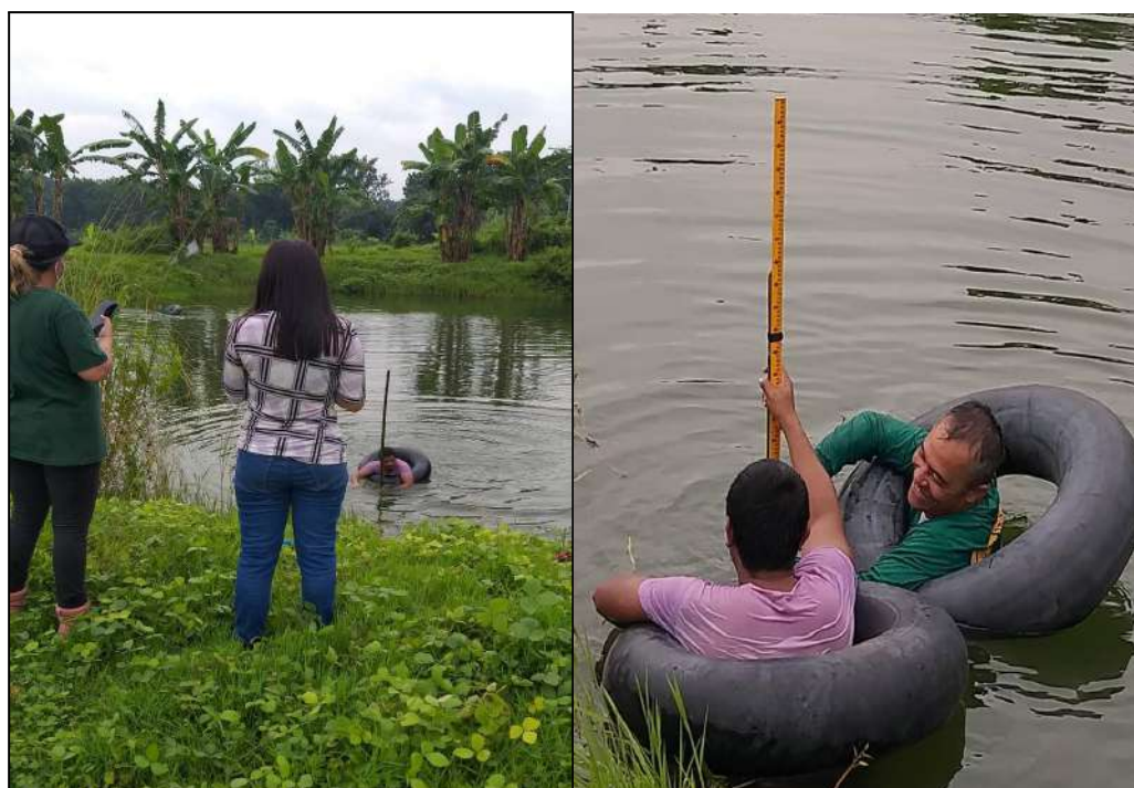
Figure 12. Installation of staff gauge, data gathering and measuring the topography of pond bottom of each point in the pond at TAU Techno demo site.
