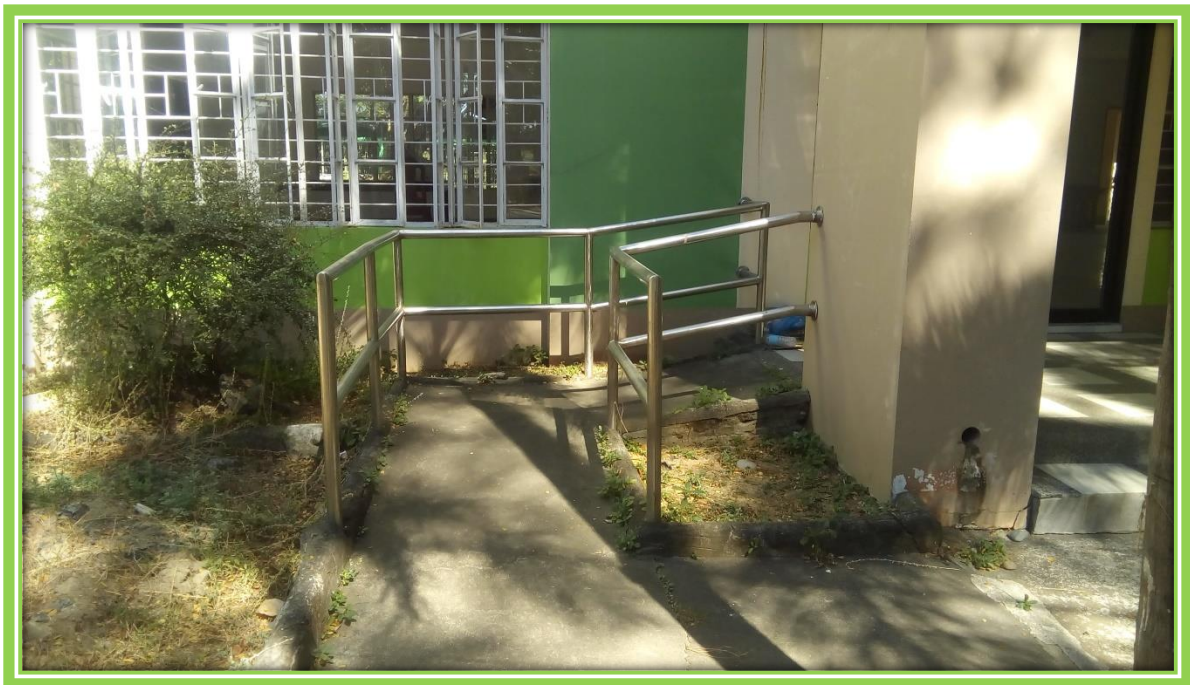
PWD Ramp at the (CEd) TLE Building
