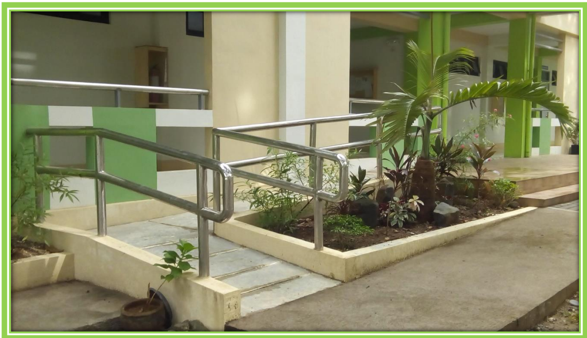
PWD Ramp at the (CEd) Home Tech. Building
