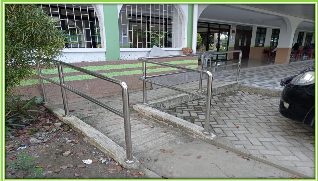
PWD Ramp at the College of Business and Management Main Building
