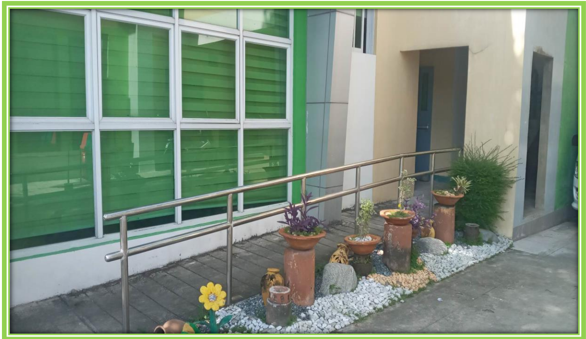
PWD Ramp at the Administration Building
