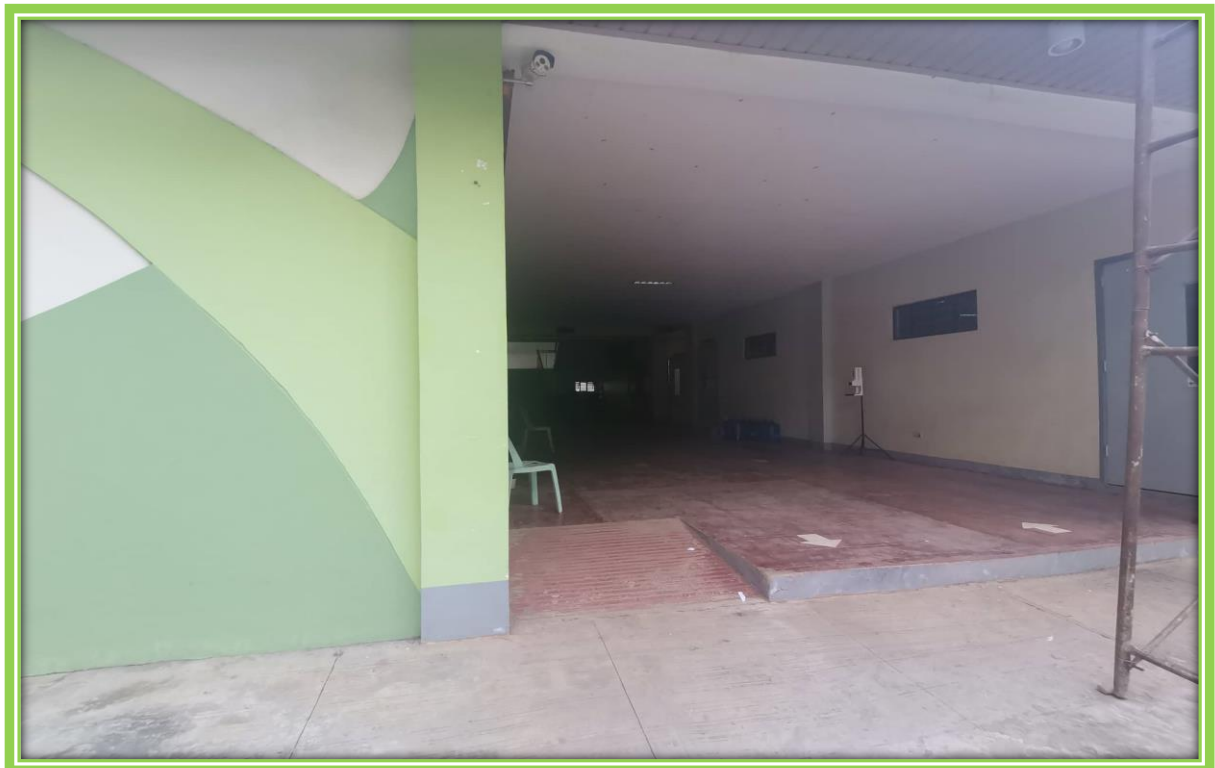
PWD Ramp at the Laboratory High School
