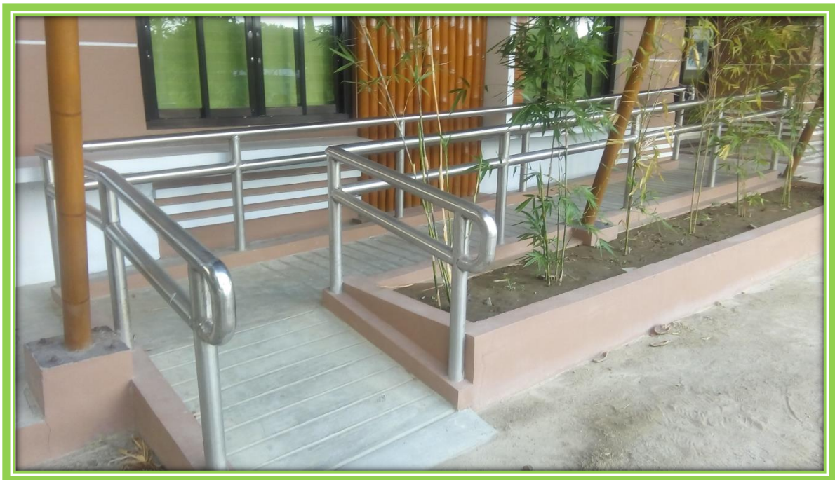
PWD Ramp at the Bamboo Training Center
