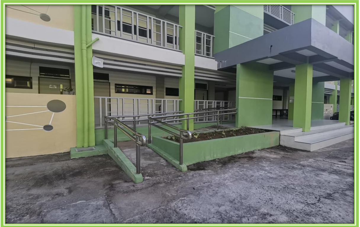
PWD Ramp at the College of Arts and Sciences Building
