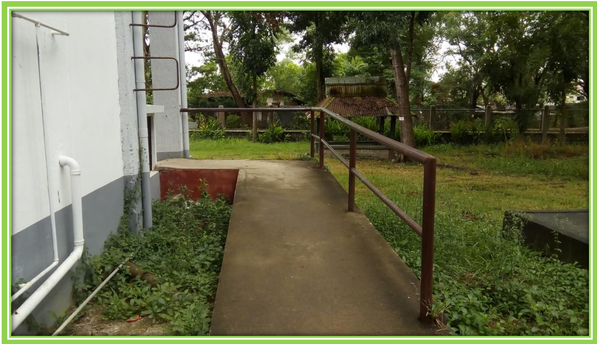
PWD Ramp at the College of Engineering and Technology (CET) Main Building
