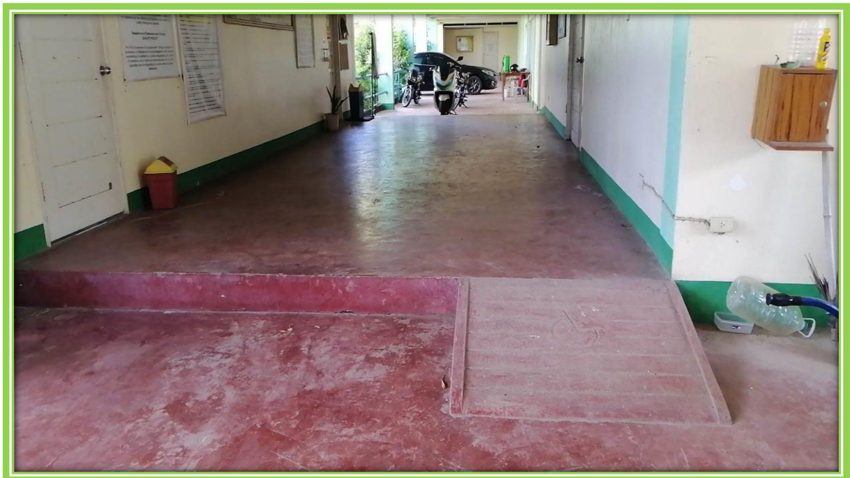
PWD Ramp at the Research and Development Building
