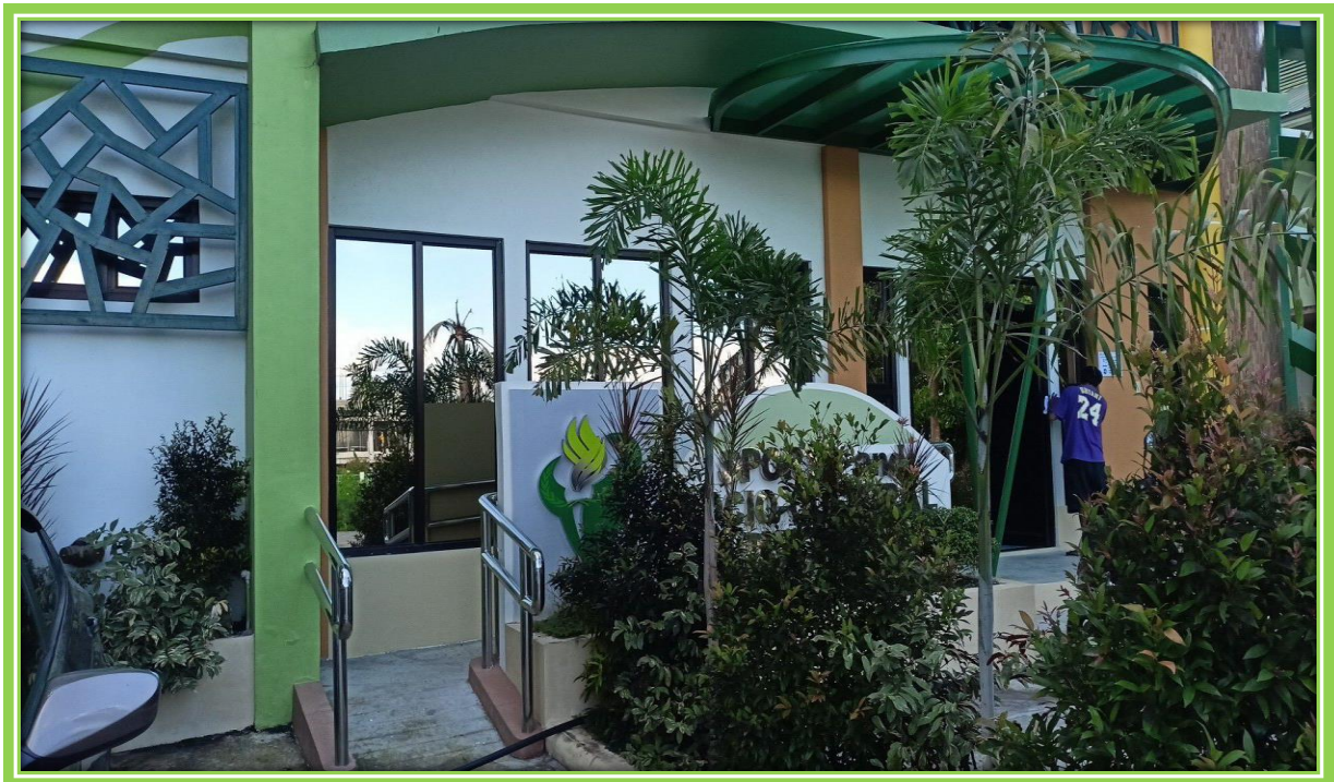
PWD Ramp at the Sports and Socio Cultural Building
