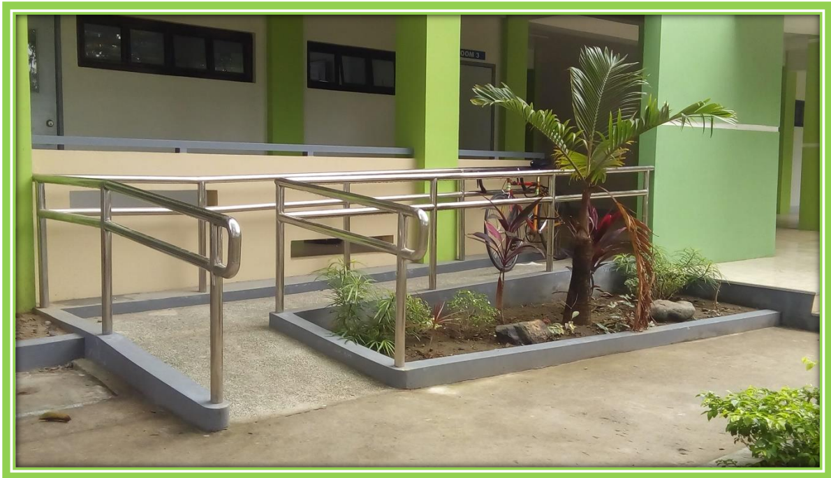
PWD Ramp at the College of Education (CEd) Gen.Ed. Building
