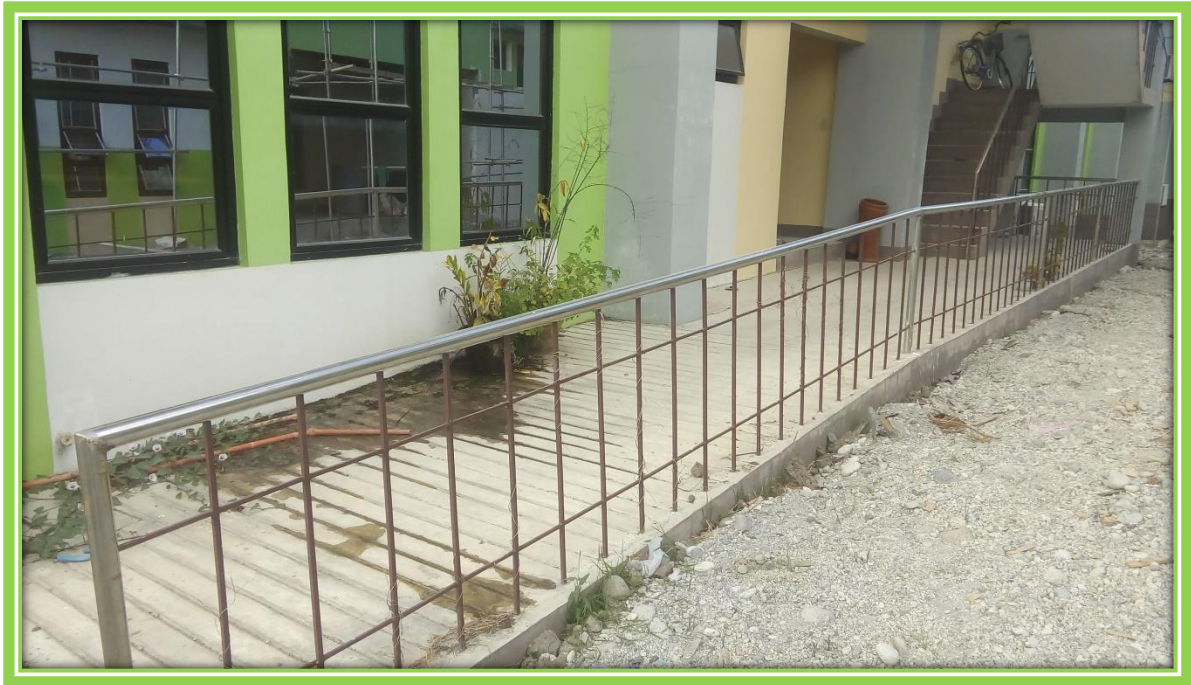
PWD Ramp at the University Library Building
