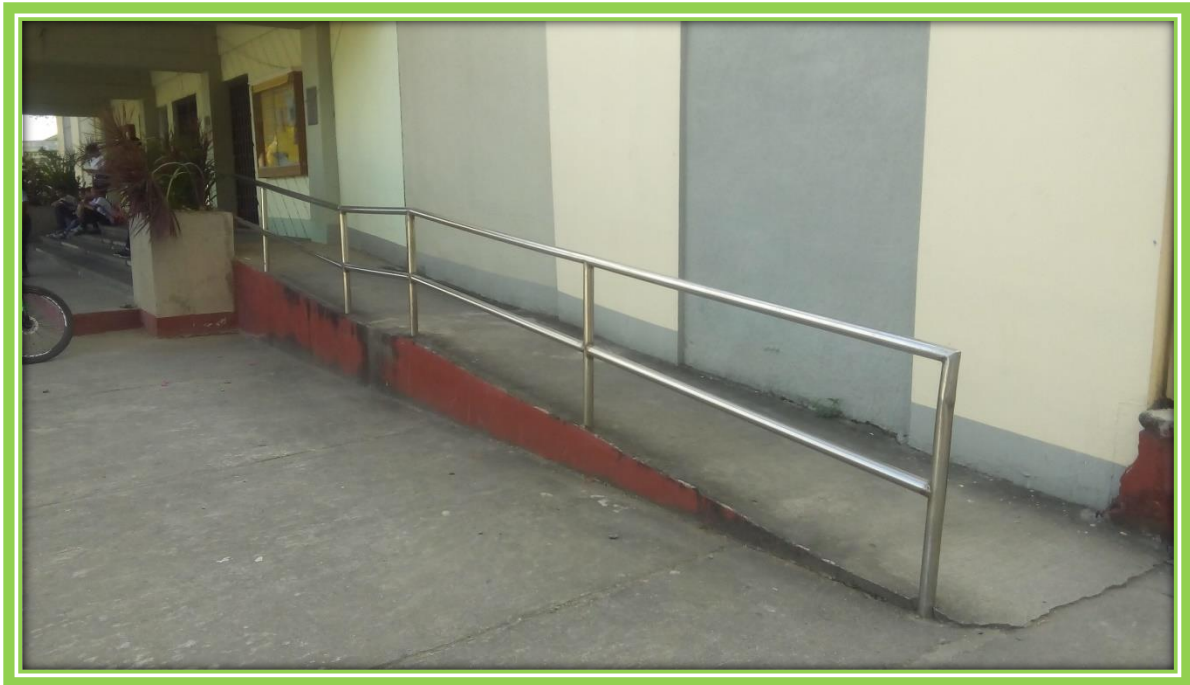
PWD Ramp at the GOT Multipurpose Center
