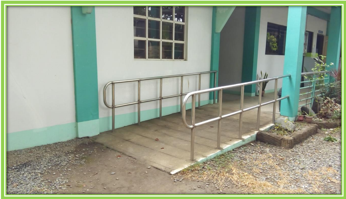
PWD Ramp at the (CEd) Ed. Tech. Building
