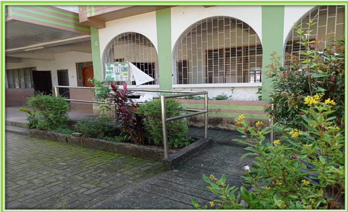
PWD Ramp at the College of Business and Management Annex Building
