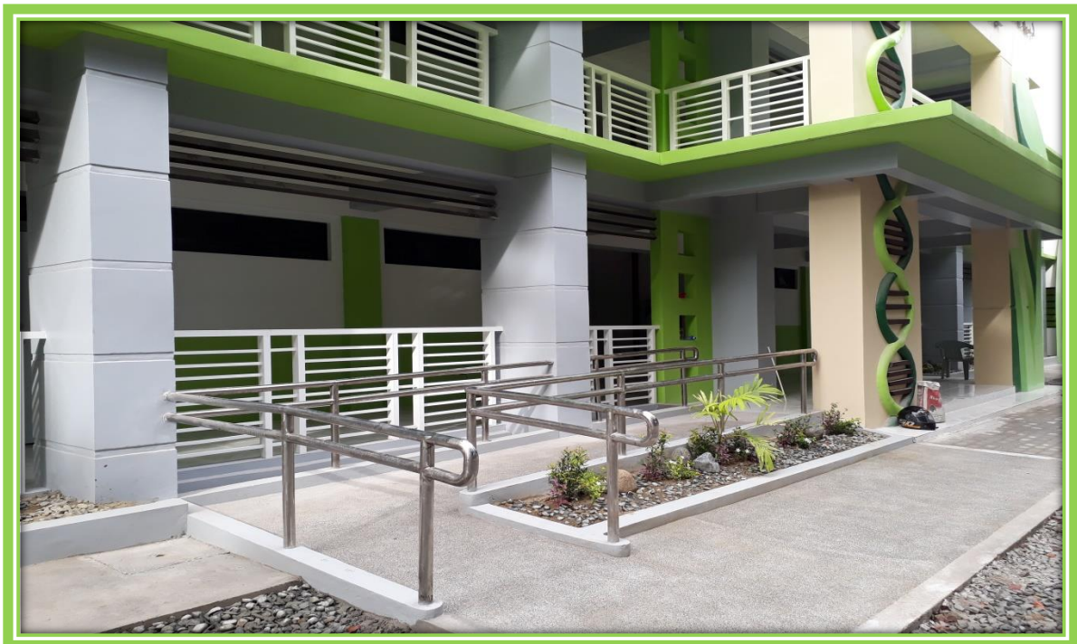
PWD Ramp at the New College of Veterinary Medicine (CVM) Bldg
