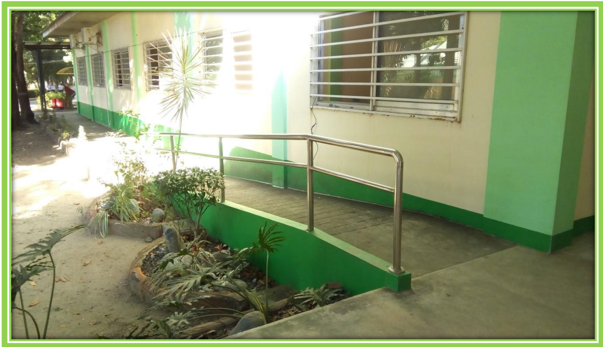
PWD Ramp at the Research and Development Building
