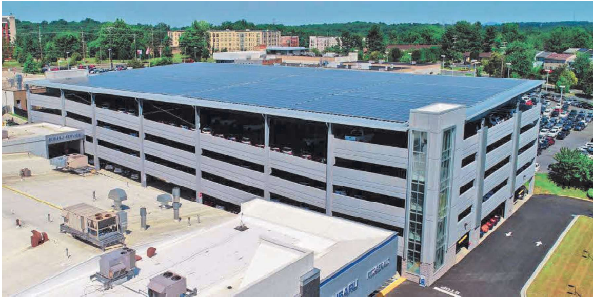
Figure 3-14: Fitzgerald Parking Garage Solar Canopy Building
