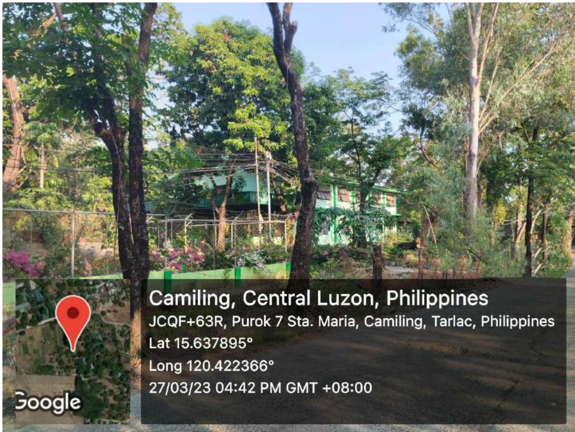
Figure 2-53: Geotagged Photo of the Student-Men's Dormitory
