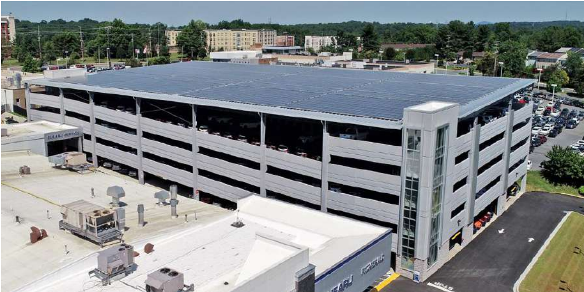
Figure 3-14: Fitzgerald Parking Garage Solar Canopy Building
