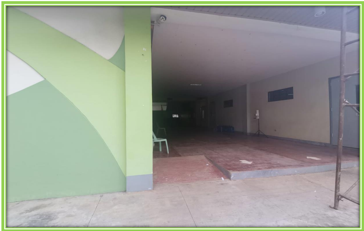
PWD Ramp at the Laboratory High School
