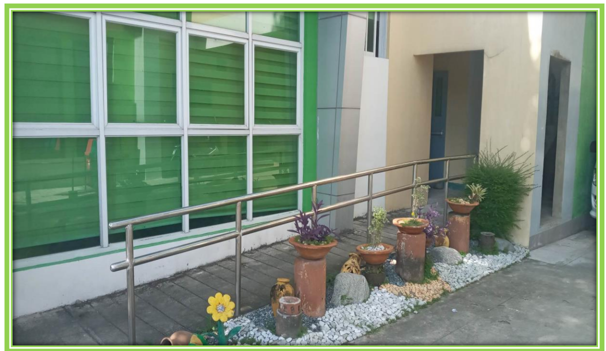
PWD Ramp at the Administration Building
