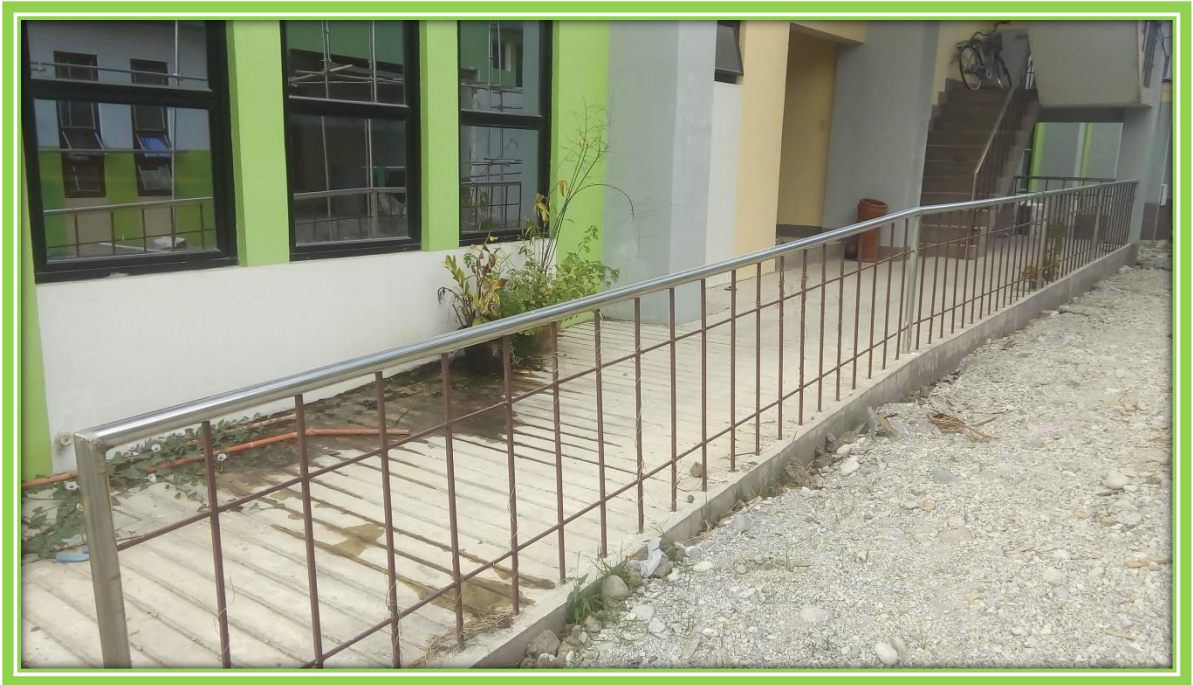
PWD Ramp at the University Library Building
