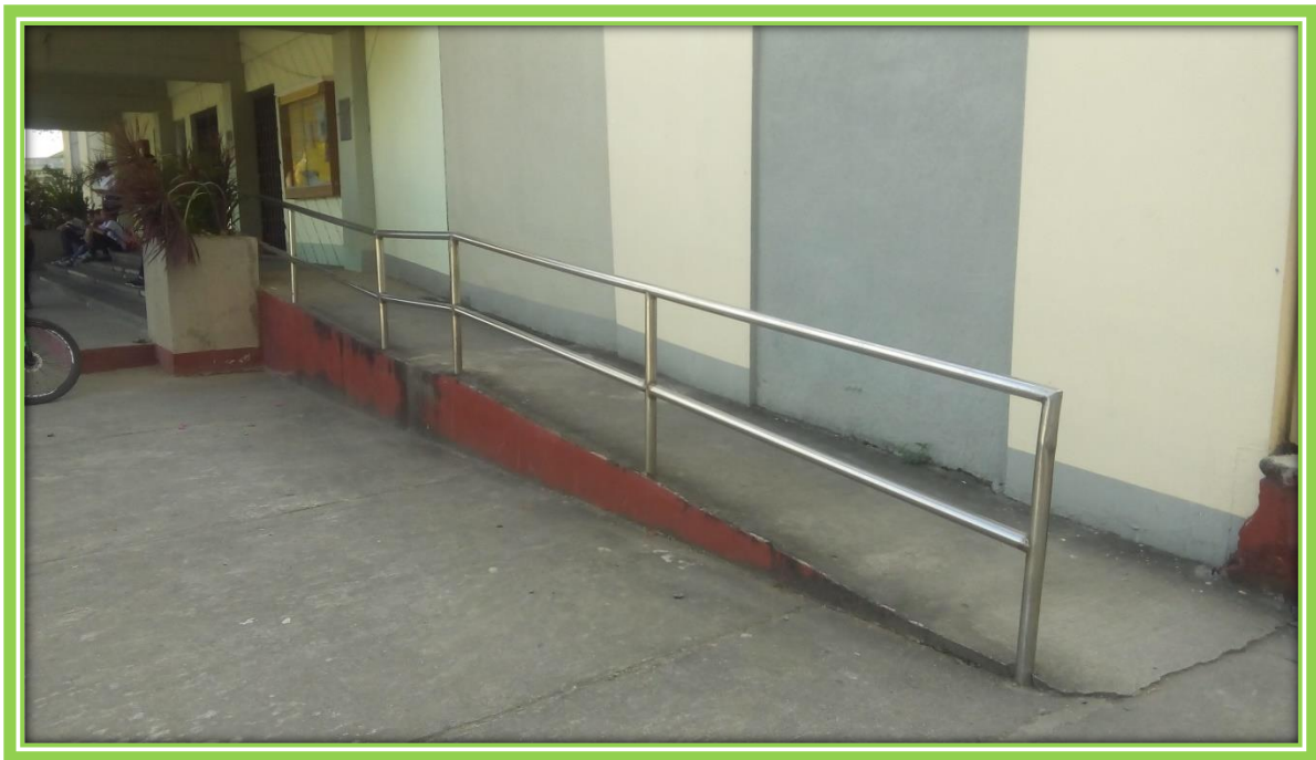
PWD Ramp at the GOT Multipurpose Center
