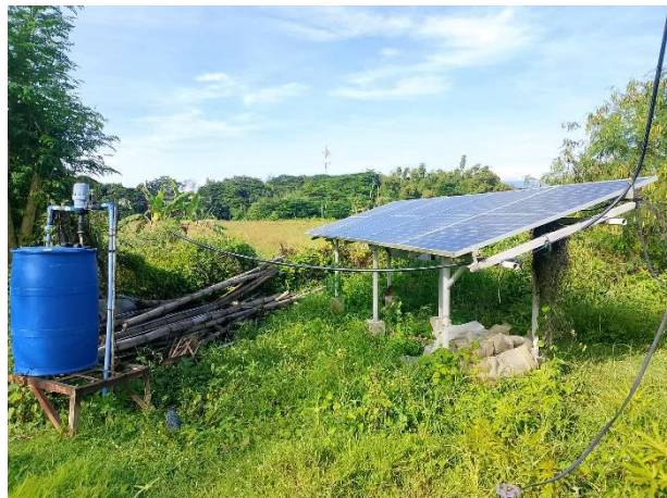
6.5.4j. Solar power-driven submersible pumps installed on dug wells and shallow wells in various locations inside the campus
