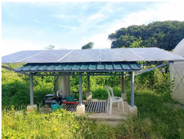
6.5.4j. Solar power-driven submersible pumps installed on dug wells and shallow wells in various locations inside the campus
