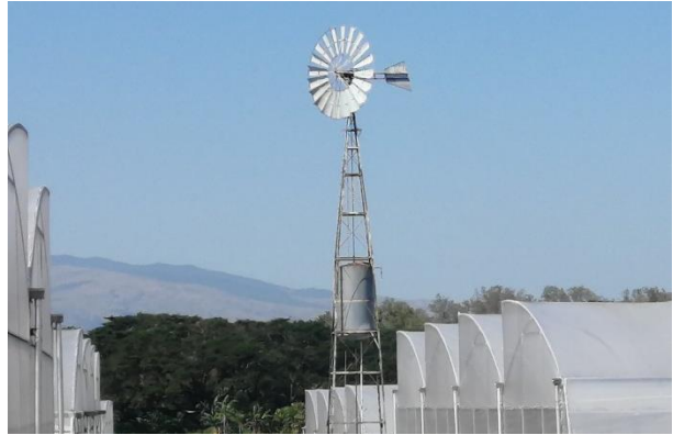
Figure 6.5.4k. Windmill-driven pumps with an elevated water tank.
