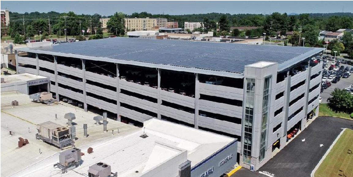
Figure 3-14: Fitzgerald Parking Garage Solar Canopy Building
